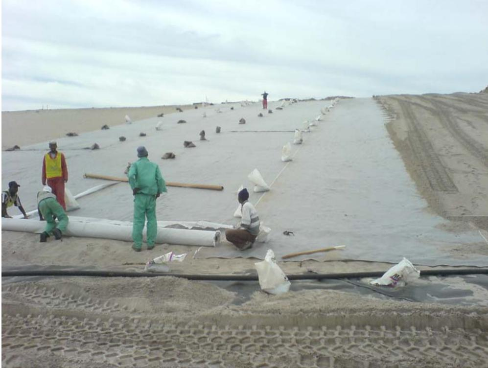
**Photo 1 : Installing the grid.**
