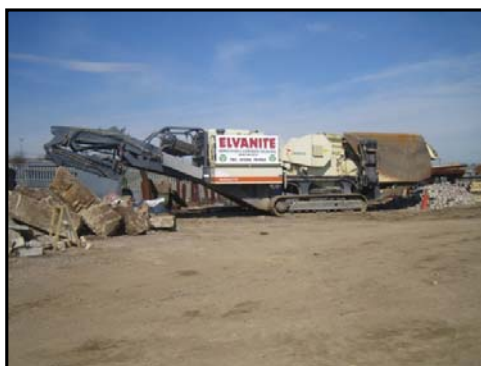
Plate 6 Mobile crusher used by Elvanite
