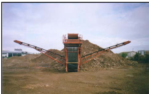
Plate 7 Screening plant on site
