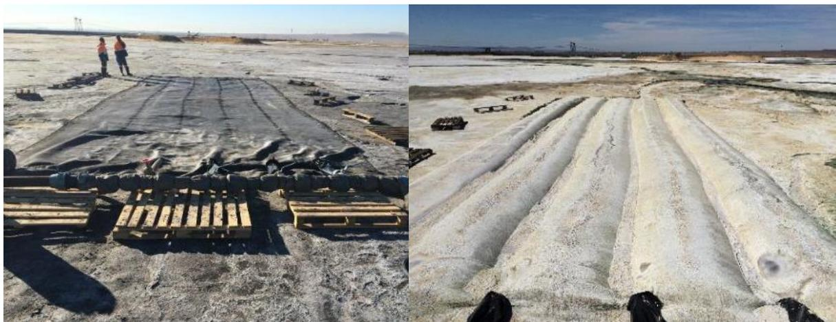
Figure 2: Installation of the trial on the horizontal surface – before and after filling.
