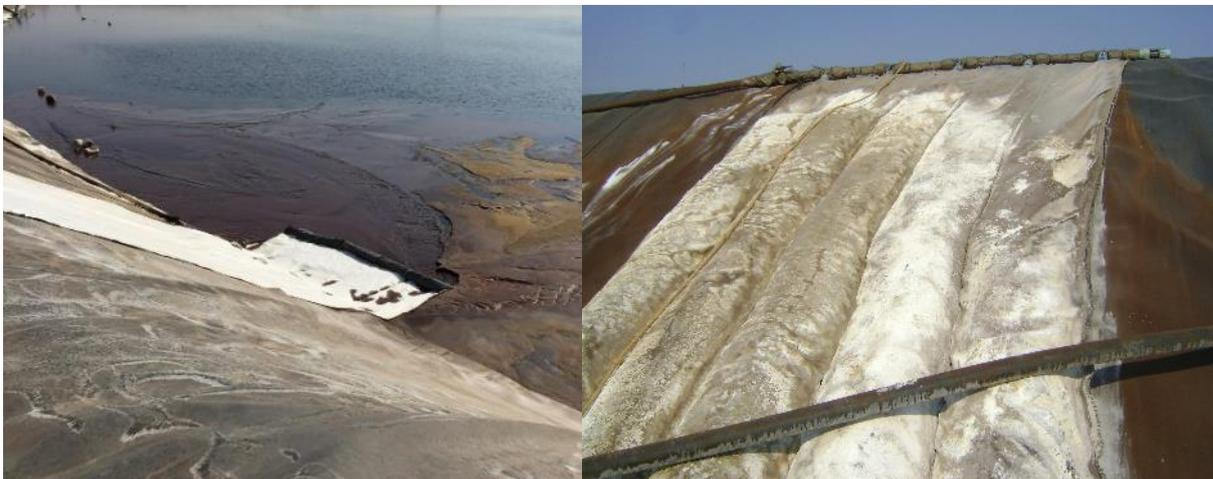
Figure 1: Installation of the trial bag on the side slope – before and after filling
