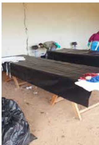
Photo 1: DPC on trestles
