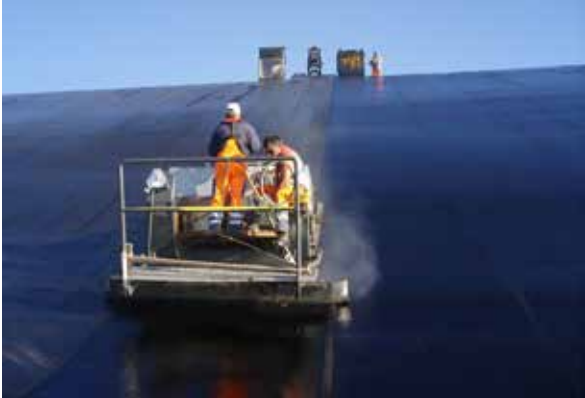
Figures 10 - Placing Mastic in the Slopes
