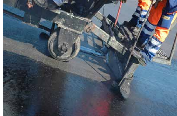
Figures 11 - Placing Mastic in the Slopes
