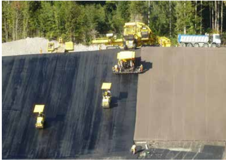
Figure 6: Finishing Phase 2 - Joint between Phases 1 and 2
