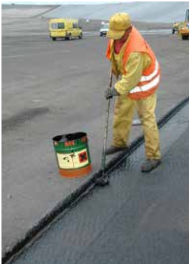
Figures 9 - Joint Preparation
