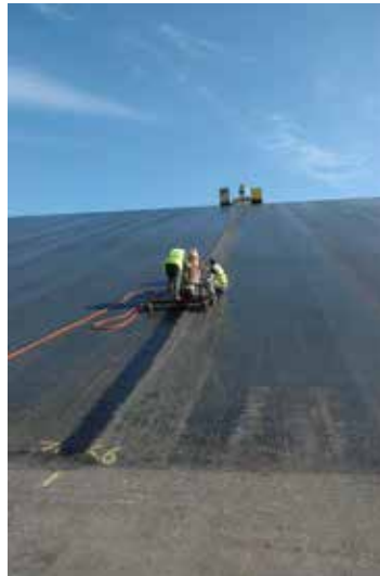
Figures 10 - Joint Re-Heating
