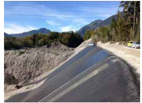
Figures 2 and 3: Construction Details of Asphaltic Layers Used at Cholwald Landfill and DAC in the Slope
