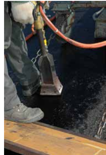
Figures 11 - Joint Re-Compaction
