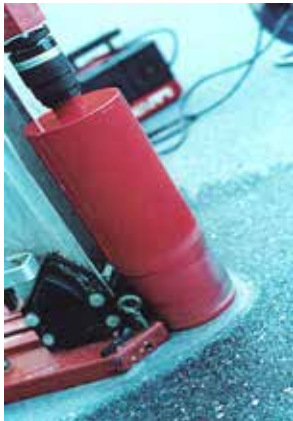
Figures 12 - Drill Cores Taken for Testing Impermeability and Vacuum Testing Joints
