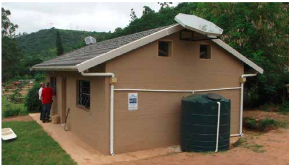
Figure 1: An example of sustainable and green low-cost housing built by USE-IT with Compressed Earth Blocks and multiple recycled components replacing conventional materials (photo supplied: USE-IT, 2012)
